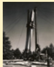
Erecting the Kensico obelisk in 1941.
